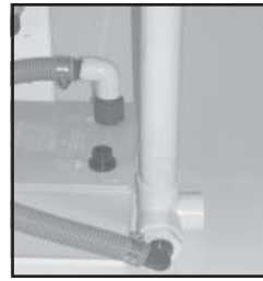
Drain tube installed
