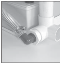
Slip-fitting inserted
