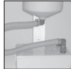
Transfer Tube installed
