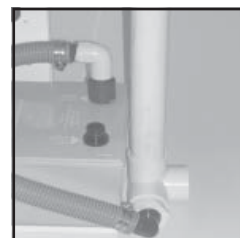
Drain tube installed
